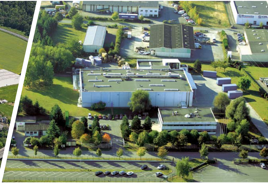
Ardrex® production plant in Soissons, France
